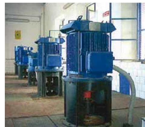
Palude Lauro drainage system. Pump room (Lesina countryside) - electric engines and inverter.
