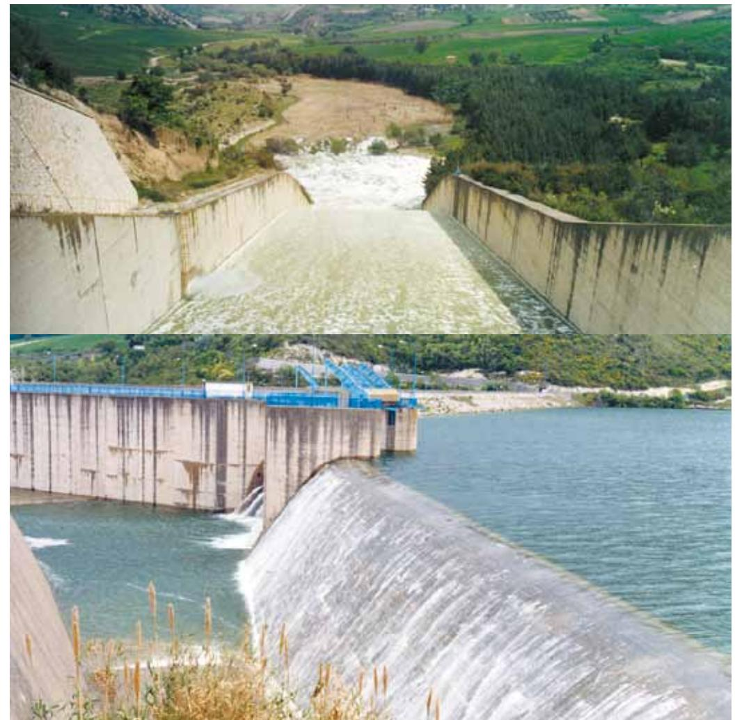
Surface discharge of Occhito dam: slide and fixed threshold.
