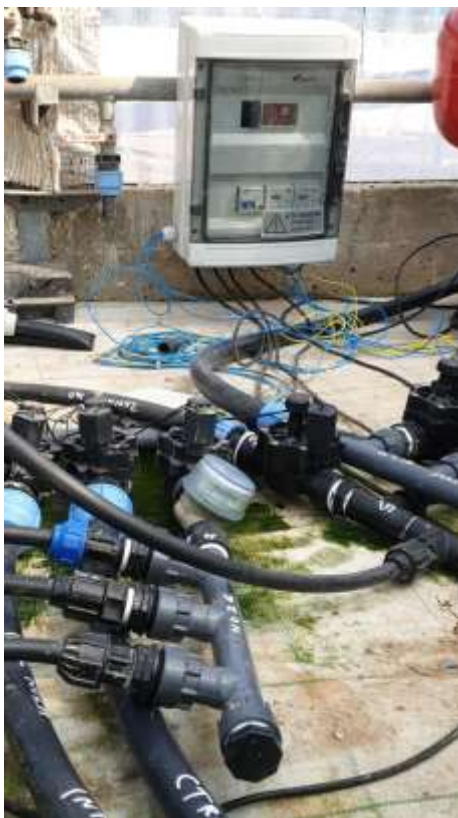
The GICK2 system connected to devices (solenoid valves and pipes) for automatic irrigation
