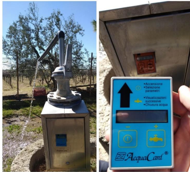
Fig. 6. Electronically fed hydrant, Sinistra Ofanto irrigation scheme.
